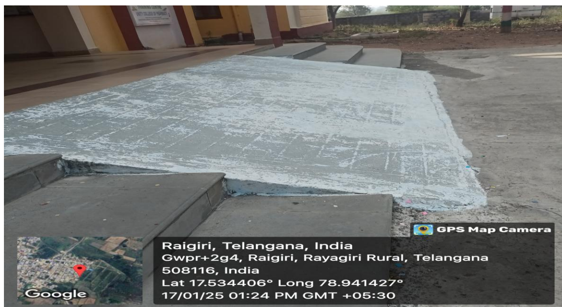
Ramp for persons with disabilities (Divyangjan)
